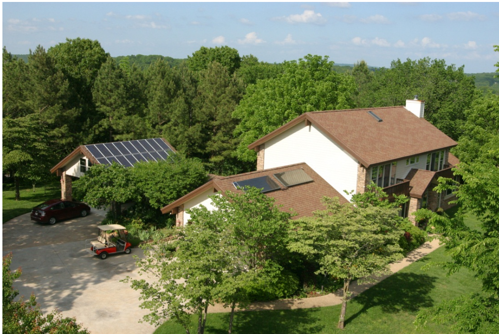
Photograph courtesy of Stitt Energy Systems, Inc., Rogers, Ark.
